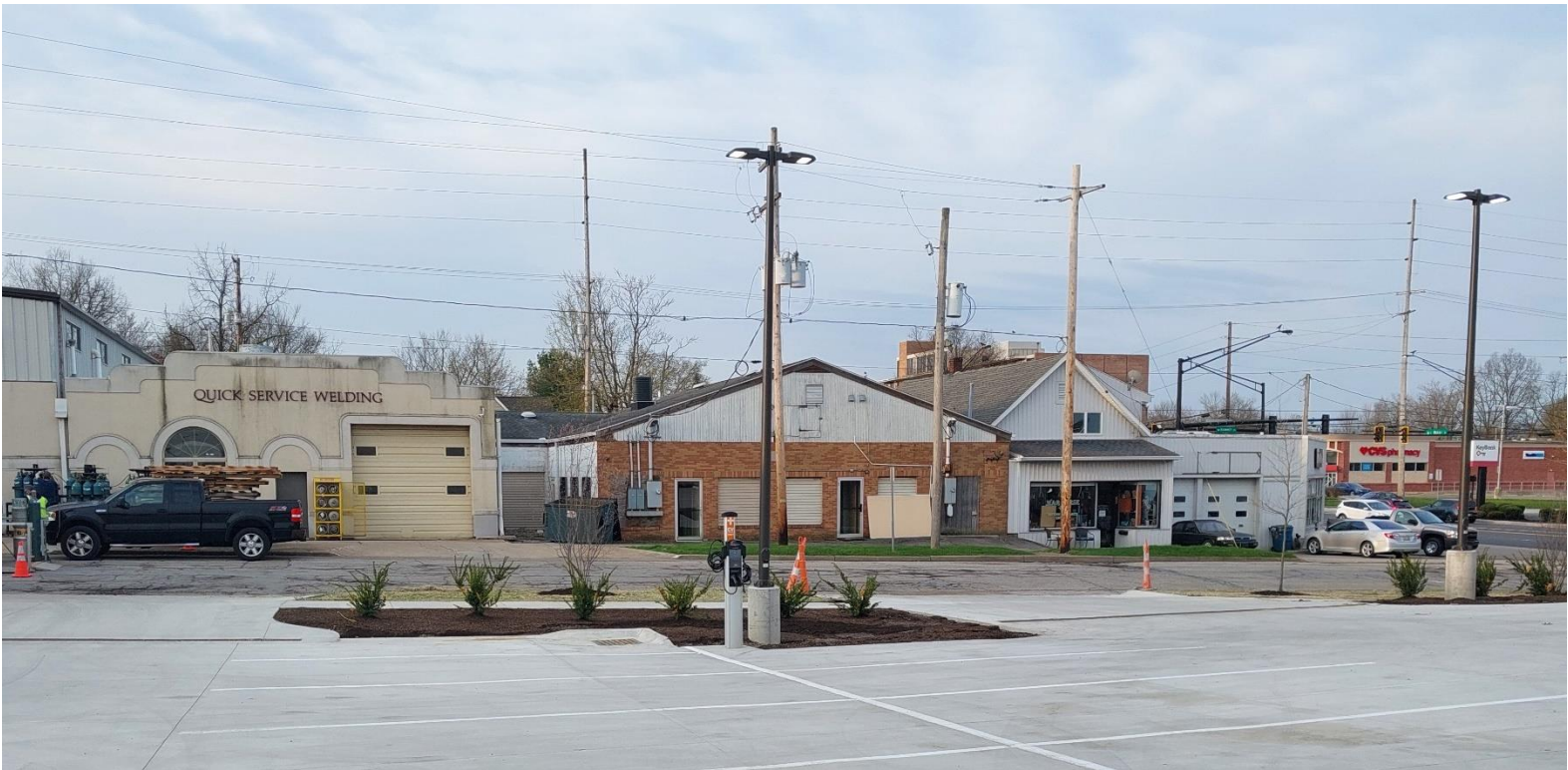
Kent City Hall EV Charging Station South-Side
